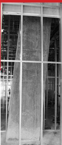
Even the support structure for the new building required a specialized design. The foundation for Armistead prevented the support columns for HBSB II from being vertical, so they were instead installed at an angle. The columns are just as sturdy and will be unnoticable when the building is complete.
